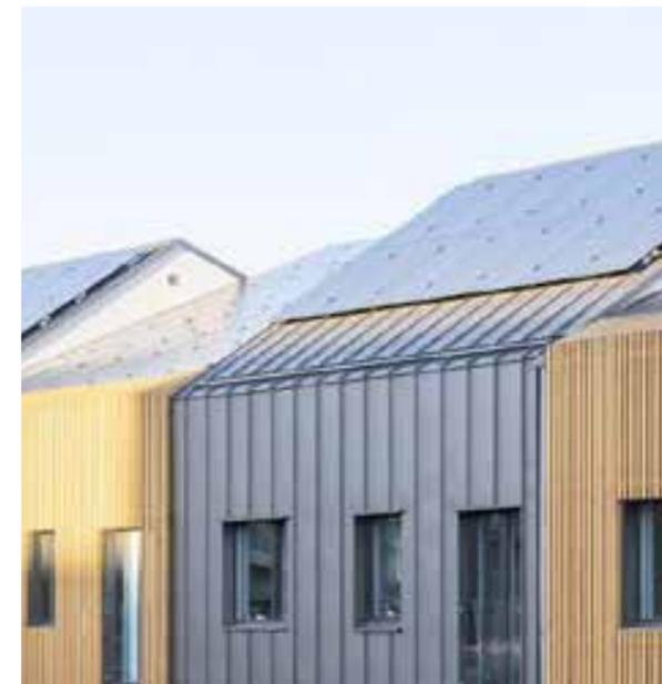
Figure 58: PV cells on pitched roof
